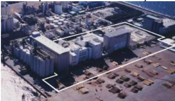
<Photo caption> Current view of Chiba Mill (white line indicates the post-expansion plant site)
