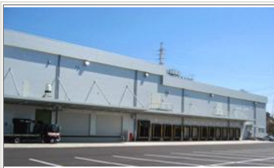
▲ Fast Foods Nagoya Co., Ltd., Kuwana Plant
