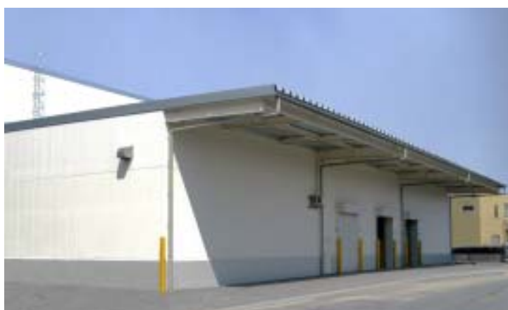
▲ Recently completed plant
